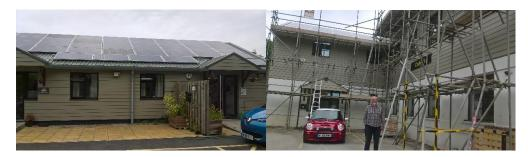
Having satisfied the Local Authority with an up-market bat-house (the building of course had bats, and they needed protection,) John and Shirley started on the factory building. It was substantially rebuilt with a timber frame, allowing for 300ml of insulation throughout, a mix of sheep wool and hemp fibre. All windows were replaced with triple-glazing. The cold store for the nuts was given a 6" concrete floor over 6" of insulation.
